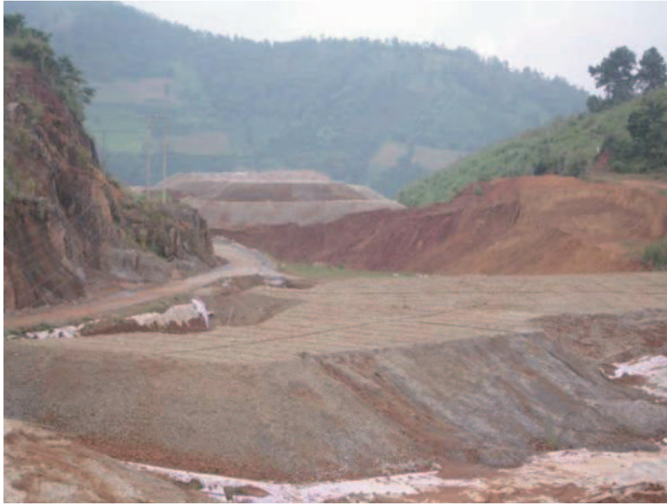
Figure 3.2 – Guoyan Gold Leach Pad
