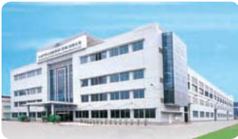
Monforts Fong's Manufacturing Plant, Shenzhen, China
