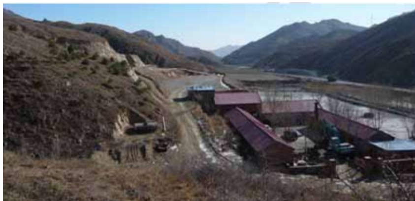
Figure 8-4: Overview of Current Processing Plant and New Concentrator Site
