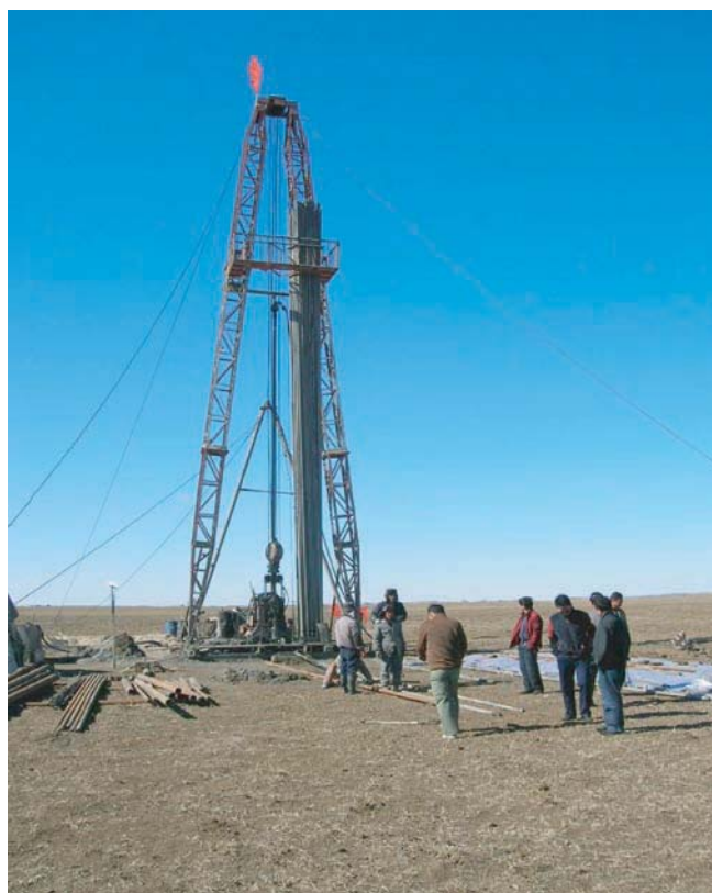
Figure 11-1: SRK Inspection of Bayanhushuo Well Site H4-4
